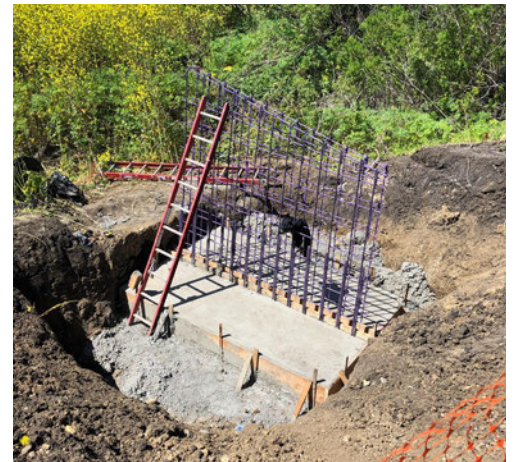
Photo taken April 2019 of construction of footings for one of the bridges of Paradiso's driveway.
